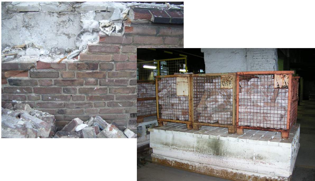
Figure 5: Whole brick recovery from masonry debris, on a semi-practical scale
